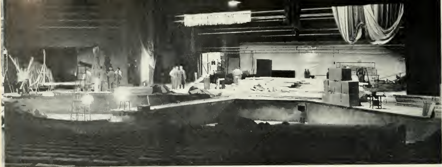
RADIO CITY'S FAMOUS CENTER THEATRE DURING CONVERSION INTO WORLD'S LARGEST TELEVISION STUDIO.
