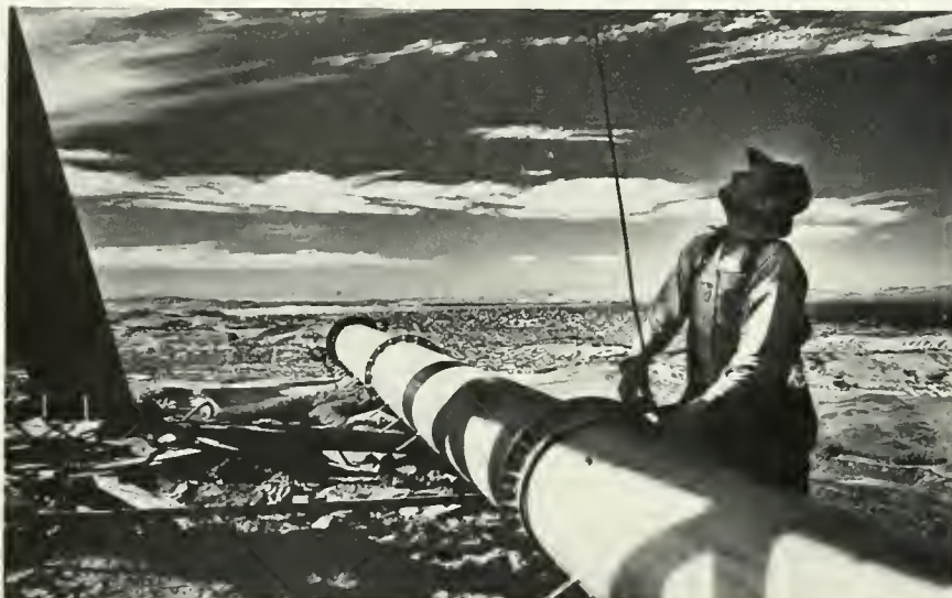
PYLON ANTENNA OF KNBC'S FM STATION ABOUT TO BE LIFTED INTO POSITION ATOP SAN BRUNO MOUNTAIN, HIGHEST POINT ON THE PENINSULA.
